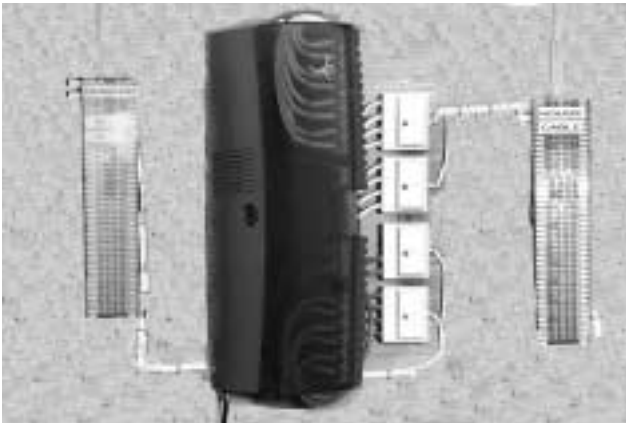
Figure 1. Example of a Single Switch Installation
