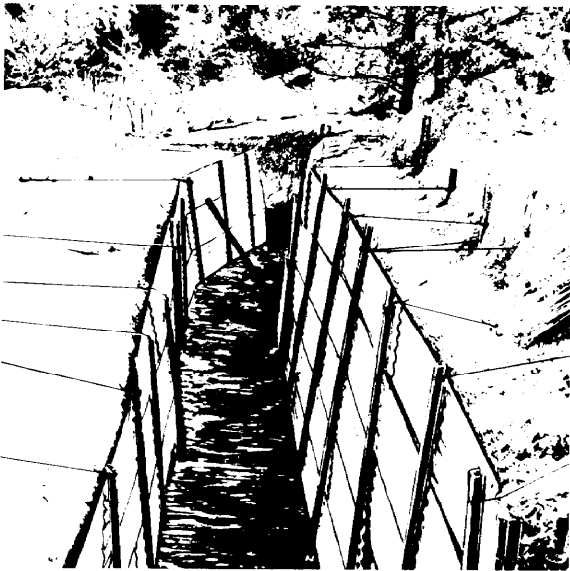
Corrugated metal sheets
