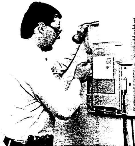
2. Route each outside line cord, one at a time, through the cable clips, located on the left side - down and across the bottom of the KSU, and on to the distribution block.
